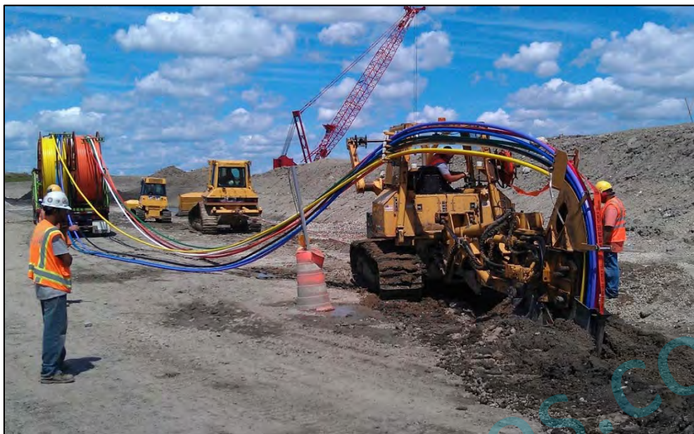
Figure 9 Example of Vibratory Plowing of Conduit
