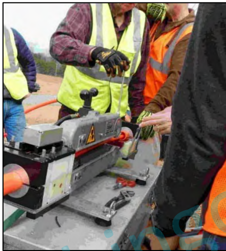
Figure 18 Jetting Microduct
