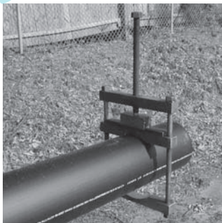
Figure 15 Mechanical Re-Rounding Clamp Installed
