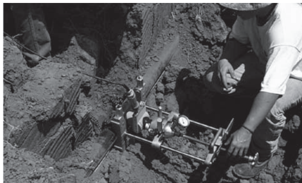
Figure 3 Saddle Fusion Repair
