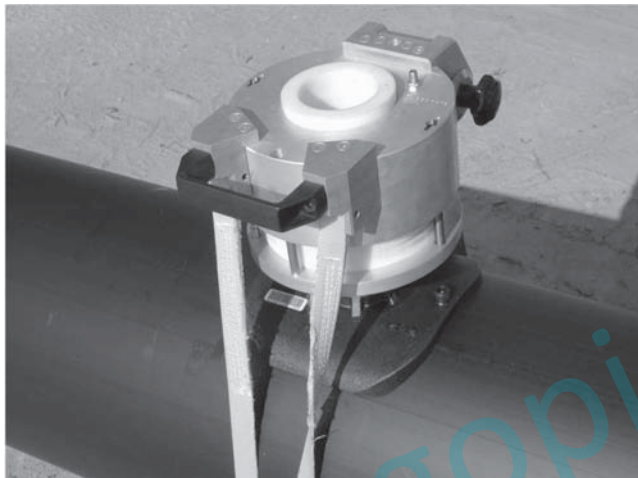
Figure 4 Electrofusion Patch Repair
