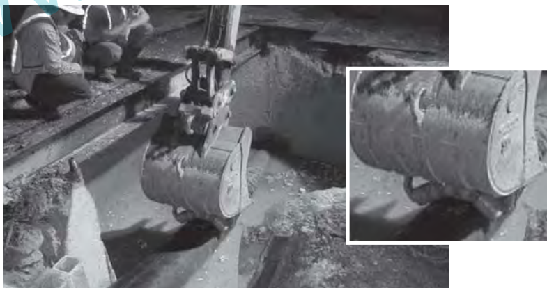
Figure 23 Protecting the PE Pipe from Groves Using Welded Wheels on the Bucket
