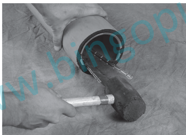
Figure 12 Install Split Ring Stiffener in PE Pipe
