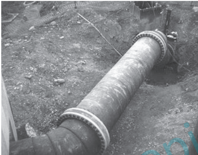
Figure 13 Flange Adapter Assembly
